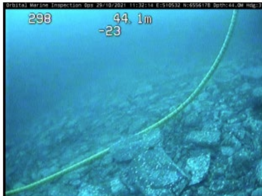
Figure 72. Typical Orbital O2-X Subsea Cable Slack
