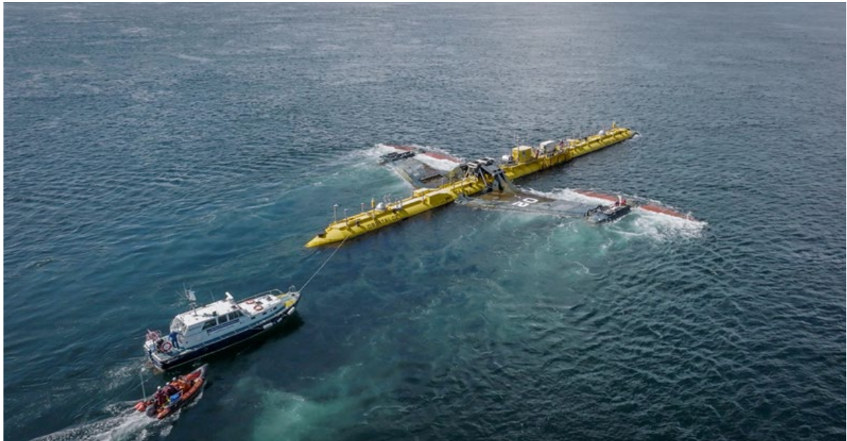
Figure 73. Example of Vessel and Boat Installing Orbital Tidal Device
